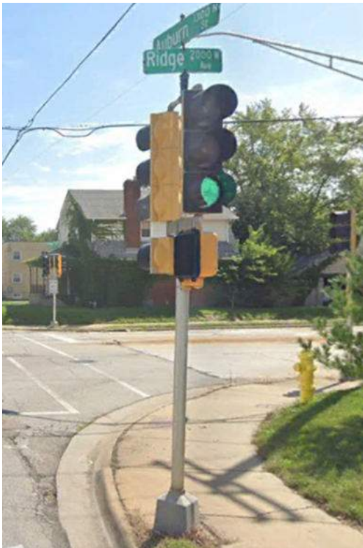
Figure 35 - Pedestal Mounted Signal at Ridge Avenue
