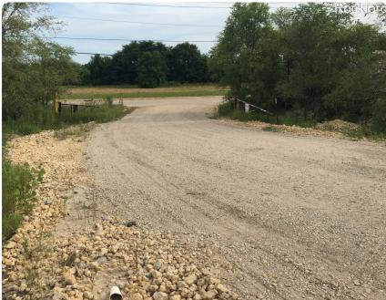
Properly installed construction entrances knock off the mud on the tires before leaving the site.
