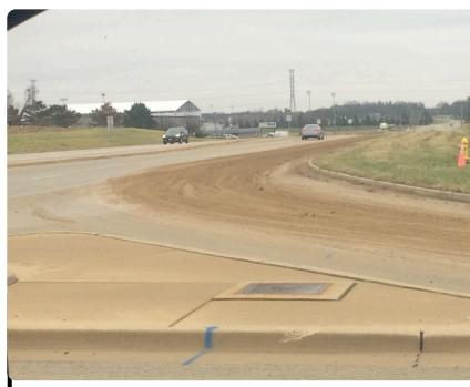
Not maintaining the construction entrance leads to tracking out sediment onto streets and is also a safety hazard to drivers.
