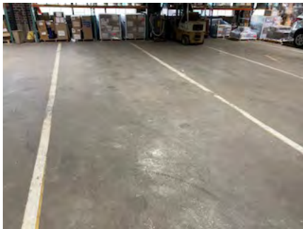
Interior Garage. Painted Floor Stripes (White and Yellow) with LBP identified.
