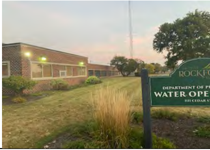
Exterior Building from Southeast Corner.
