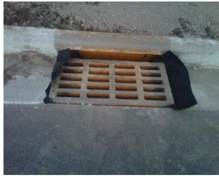
The Illinois Urban Manual does not allow fabric for inlet protection.
